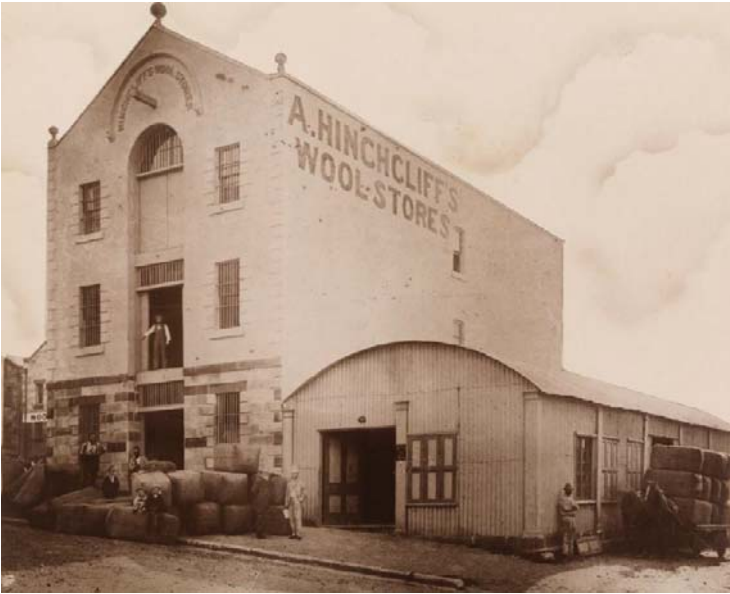
FIGURE 12 – HINCHCLIFF'S WOOL STORES, PRE-1882
