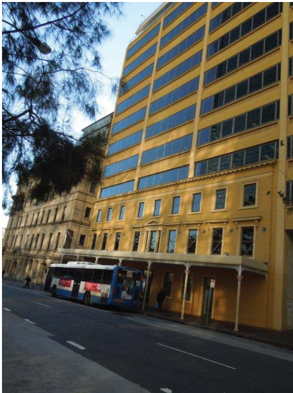
VIEW NORTH ALONG LOFTUS STREET IN THE YOUNG AND LOFTUS BLOCK. PRECINCT EXCLUDES CUSTOMS HOUSE TO THE NORTH
